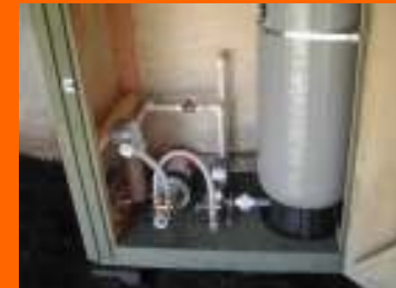
Solar Water Pumping
